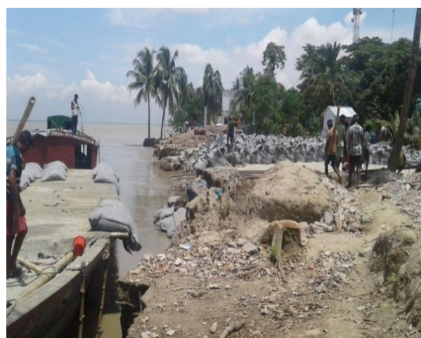
Figure 4: Dumping of sand bags by BWDB to prevent right bank erosion temporarily at Naria.
