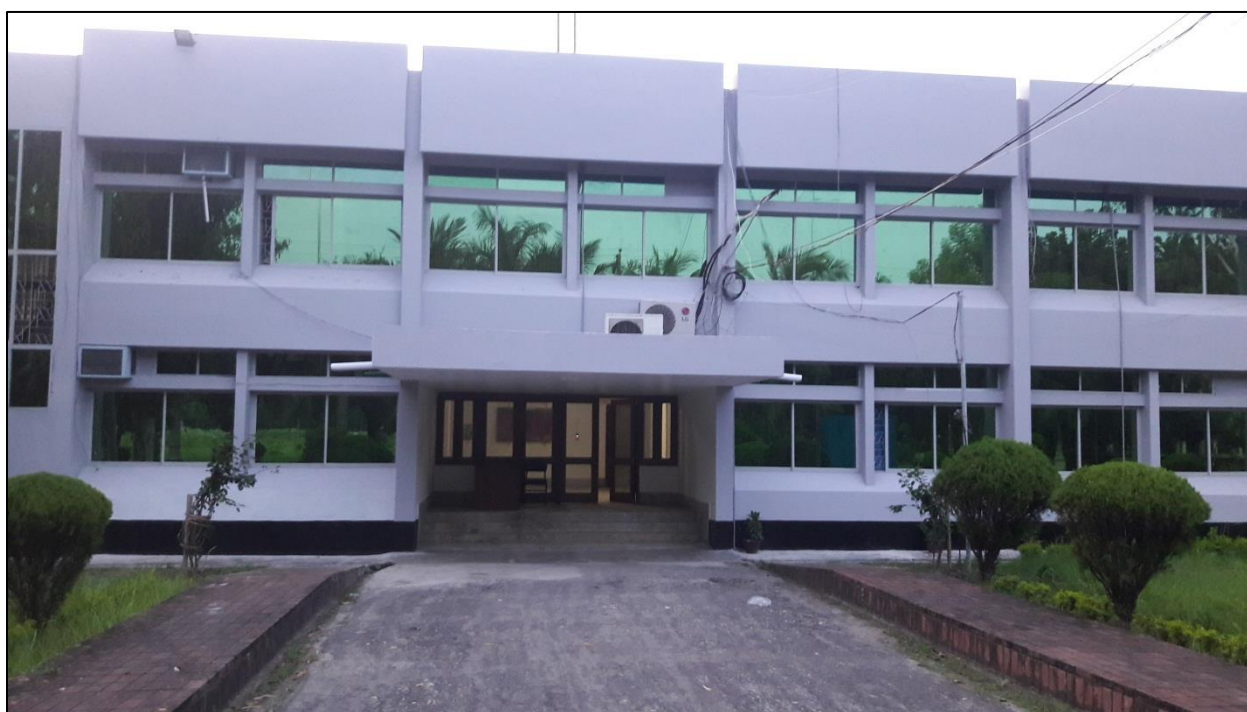
Figure: Modernization of Director General Office (Administration and Finance Building)
