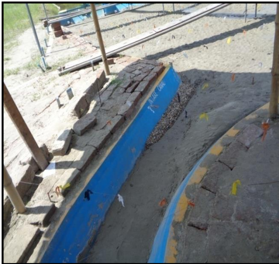
Figure 2: Launching apron at the off-take mouth along the right bank
