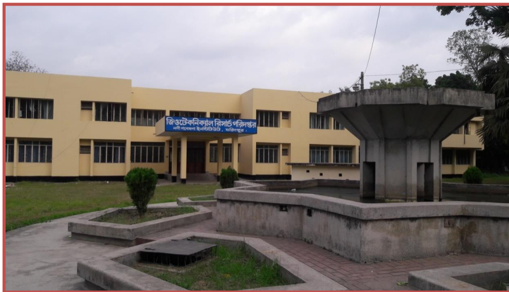
Figure: A view of Geotechnical Research Directorate Building
