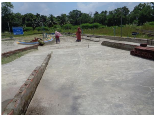
Figure 1: Routine maintenance work around the (EGB) model bed
